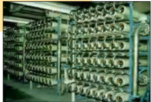
Water Factory 21 treats wastewater (left) from Orange County Sanitation District by reverse osmosis (below). More than half the injected wastewater flows inland to the potable water supply.
